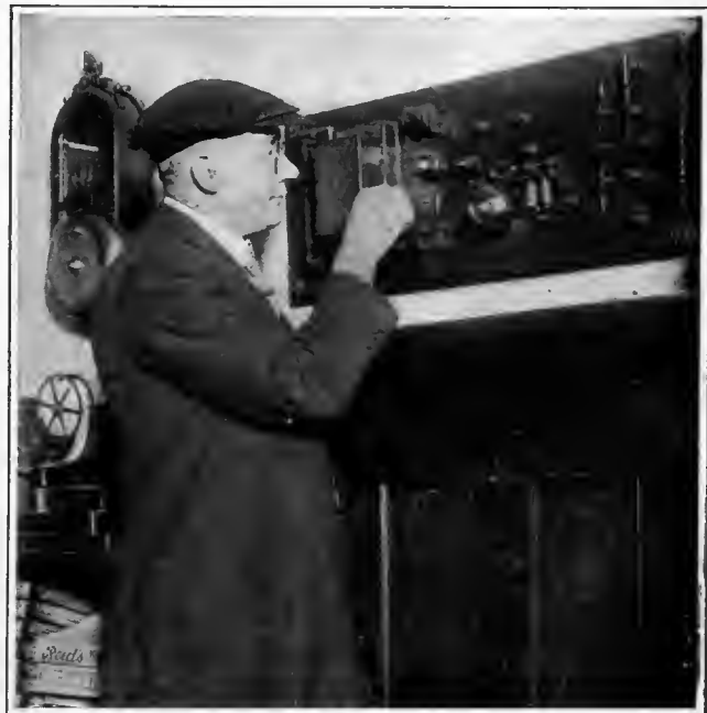
RADIO PRINCIPLES AT WORK IN THE POWER HOUSE
